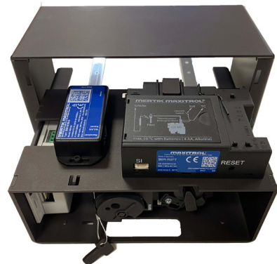
Small inspection grate – inside
