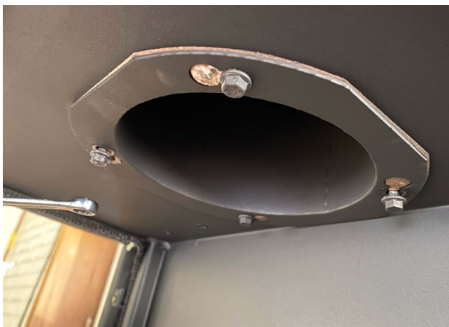
1. Loosen two of the bolts diagonally.
