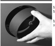
Mount the flue collar on back flue outlet hole using three M6x20 cylinder screws and M6 nuts.
