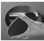
Remove any top plate, baffle plate and smoke chikane. Remove the blanking plate (3 M6 nuts) and its sealing.
