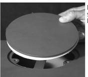
Mount the blanking plate on upper flue outlet hole - be sure to place the sealing correctly.
